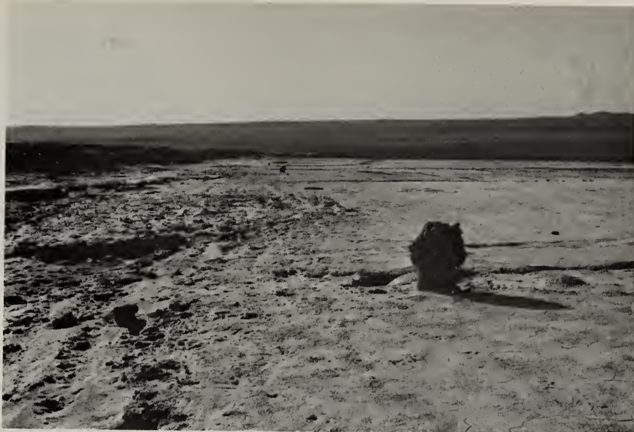
Figure 105: Stumps of telegraph poles near Kosmo (BLM photo)
